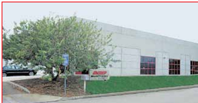
This facility is home to ARP's heat-treating operations.
